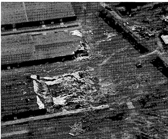
Warehouse damage in Niles included the collapse of the end of one building as the tornado clipped its edge.
