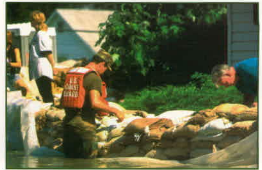
▲ Photo: Federal Emergency Management Agency
